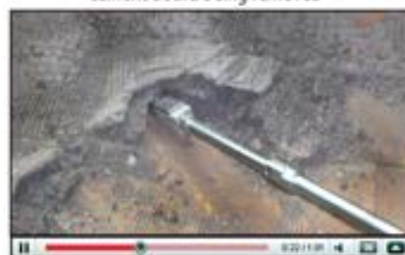
Cement board being removed
